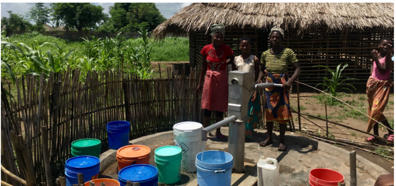
Members of Nacuta community use a water pump, which was rehabilitated after suffering significant damage during Cyclone Kenneth. Photo: Ayuda en Acción
